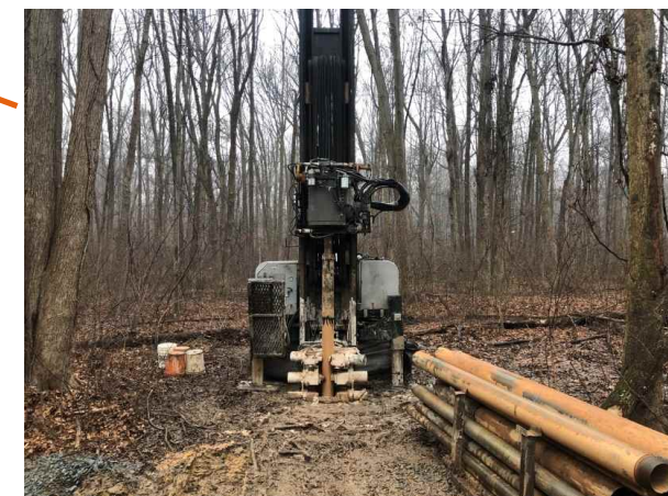
Deeper Profiling/ Well Installs in Wooded Areas (Sonic Track Rig)
