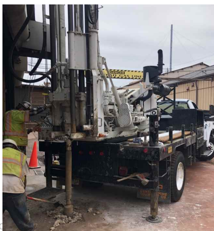
Shallow Well Installation (Hollow- Stem Auger Truck Rig)
