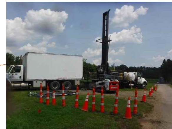
Deeper Profiling/ Well Installs in Wooded Areas (Sonic Track Rig)
