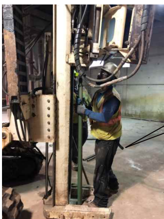
Shallow Drilling Inside Buildings (Direct-Push Track Rig)
