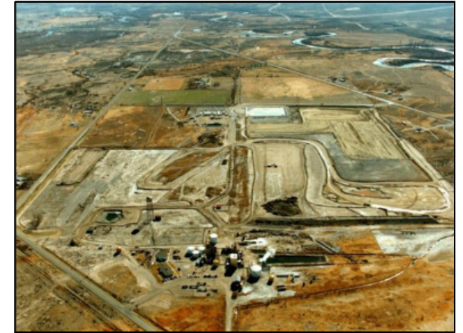
Riverton, Wyoming, Processing Site
