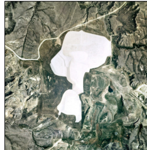
Gas Hills, Wyoming, Disposal Cell
