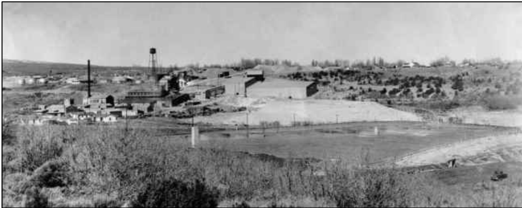
Monticello site before remediation
