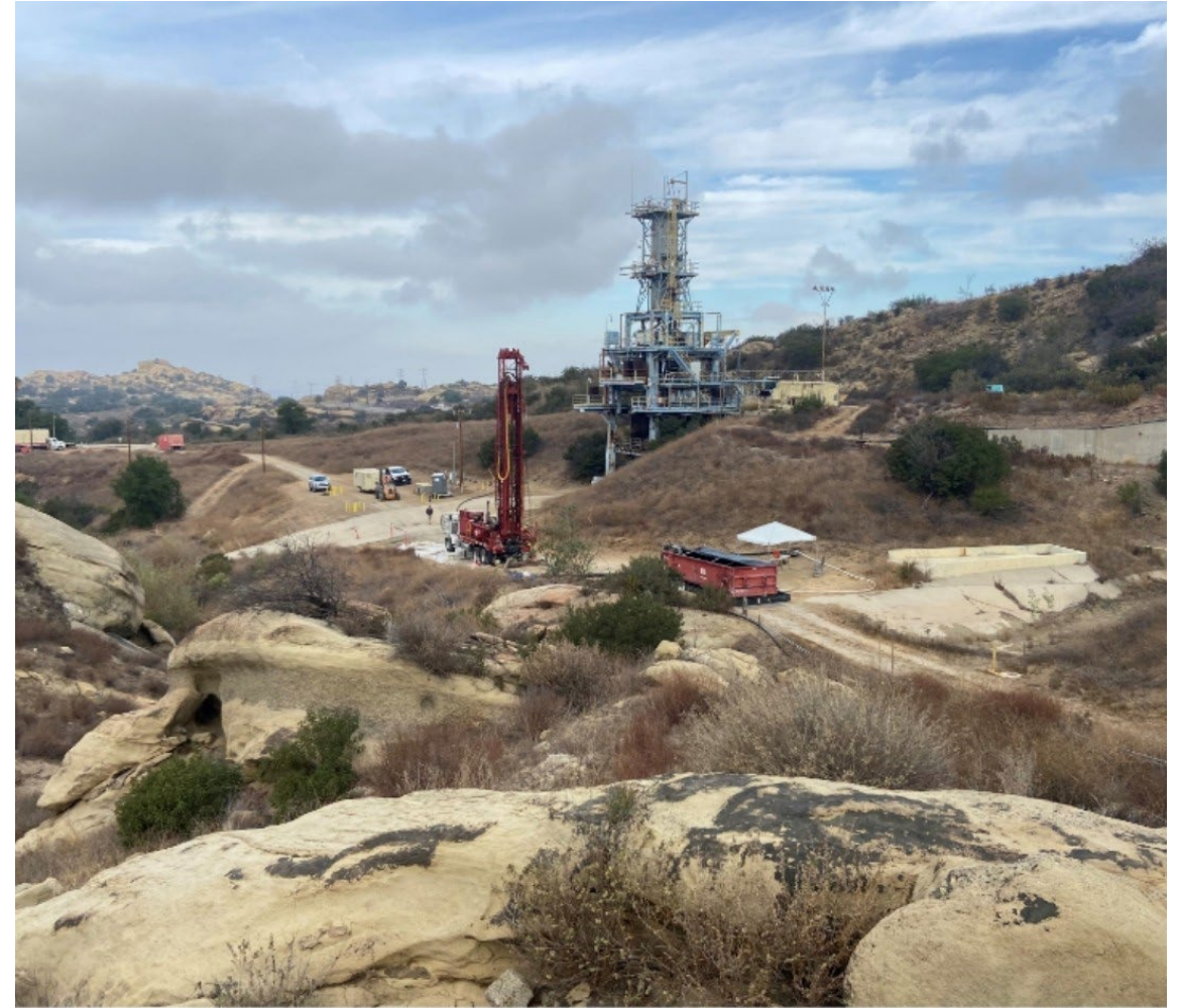
Above: Drilling of Groundwater Remediation Well
