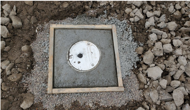
IW-001 and 002: cased to 96 and 104 feet bgs
