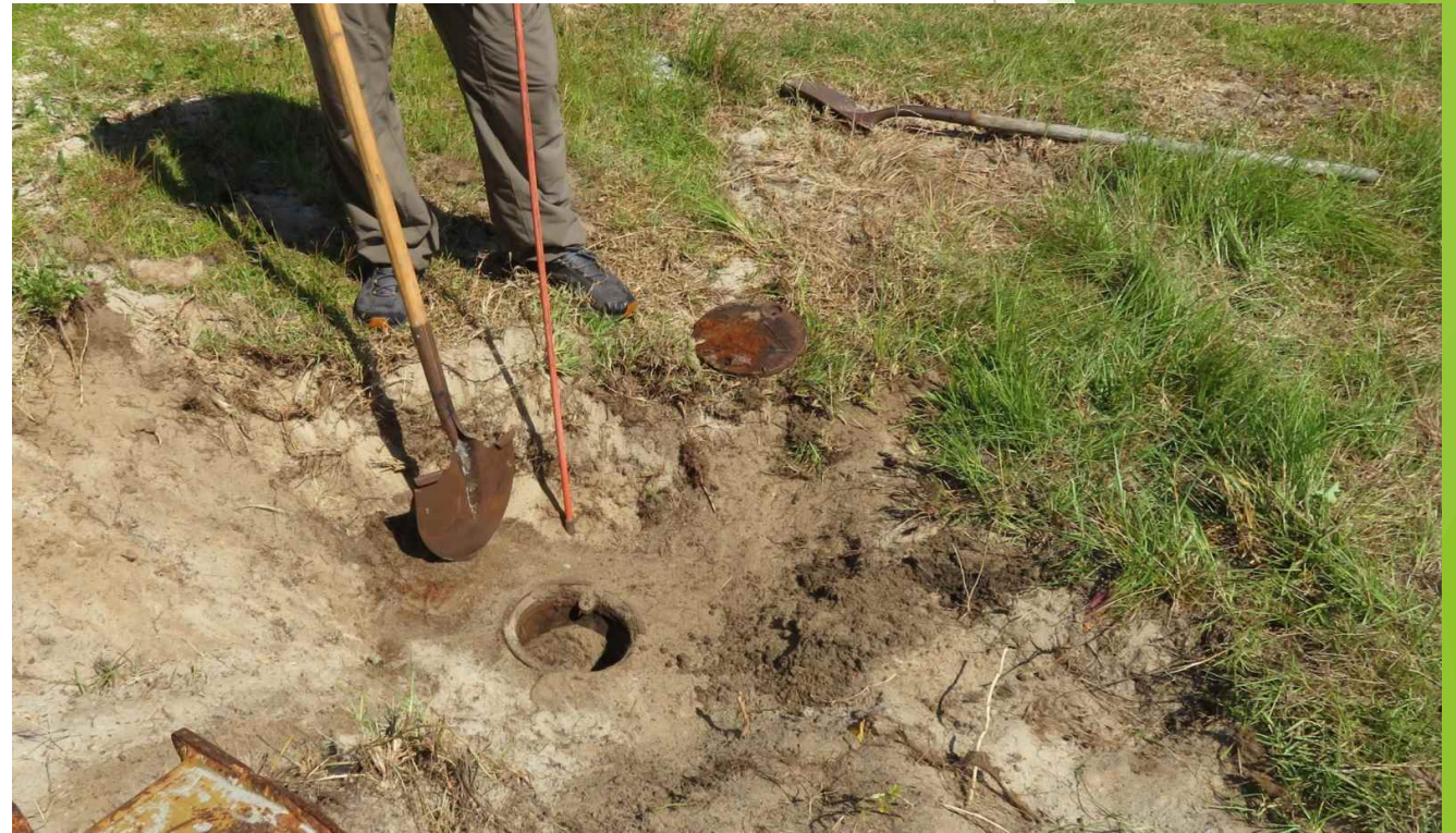
Monitoring well buried under sand
