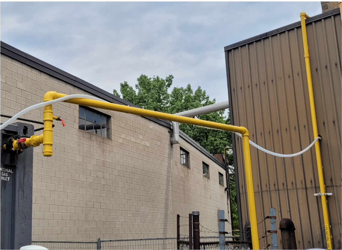
Left: Gas line which had to be re-routed for ISTR Top: Developing MPE wells Bottom: Lifting boiler up and over building
