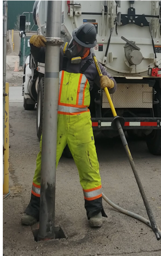
Clearance of holes by soft dig methods to 5 ft BGS
