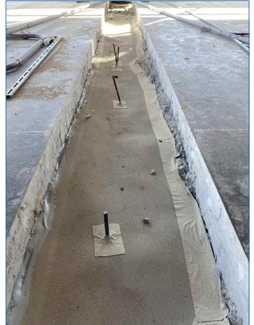
Retrofit trench to convert from passive to active
