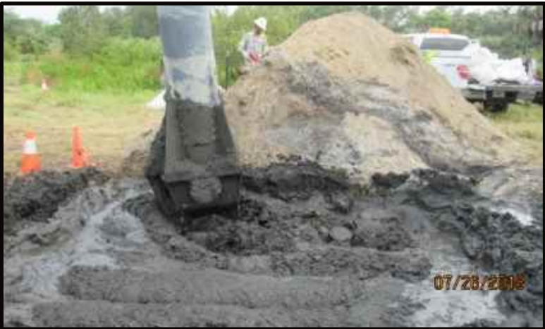
Soil Mixing with RemBind® (Test Pit 4)
