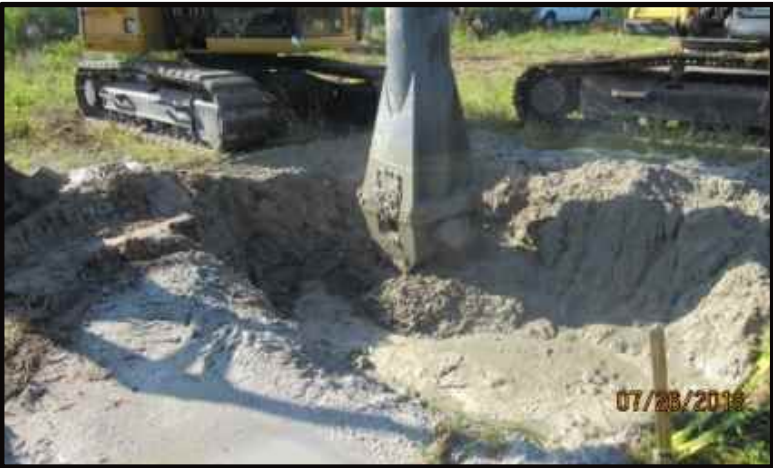
Soil Mixing with FluoroSorb® (Test Pit 2)
