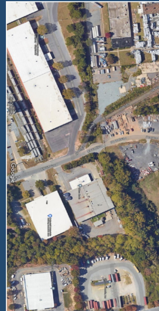
Clean Earth Charlotte Facility Aerial (courtesy Rob Martin, Clean Earth)
