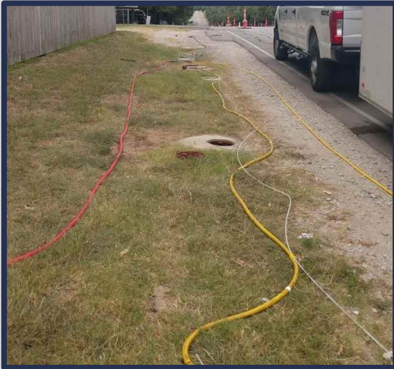
Injection lines and manifold
