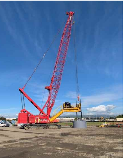
Phase 1 ISS Drilling Rig (taller mast, more torque, larger-diameter augers)
