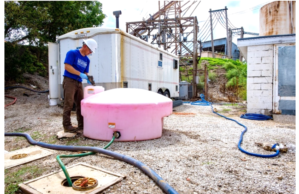
Diluted Ivey-sol in water with tracer added – pre-injection mixing.
