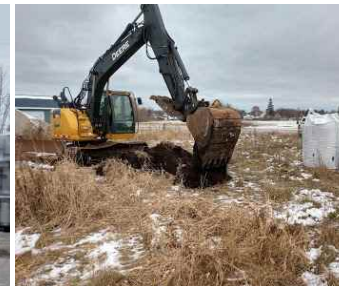
Excavator based soil mixing
