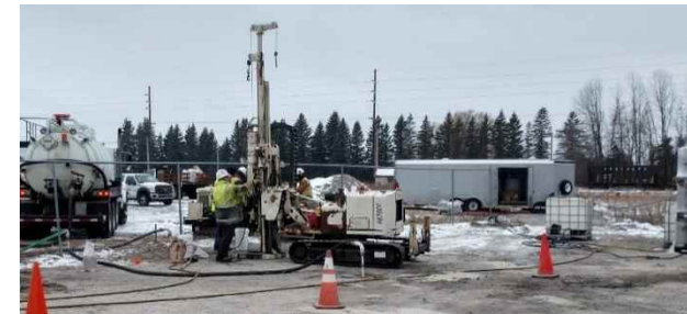
Direct Push Injection using “Push-Pull”
