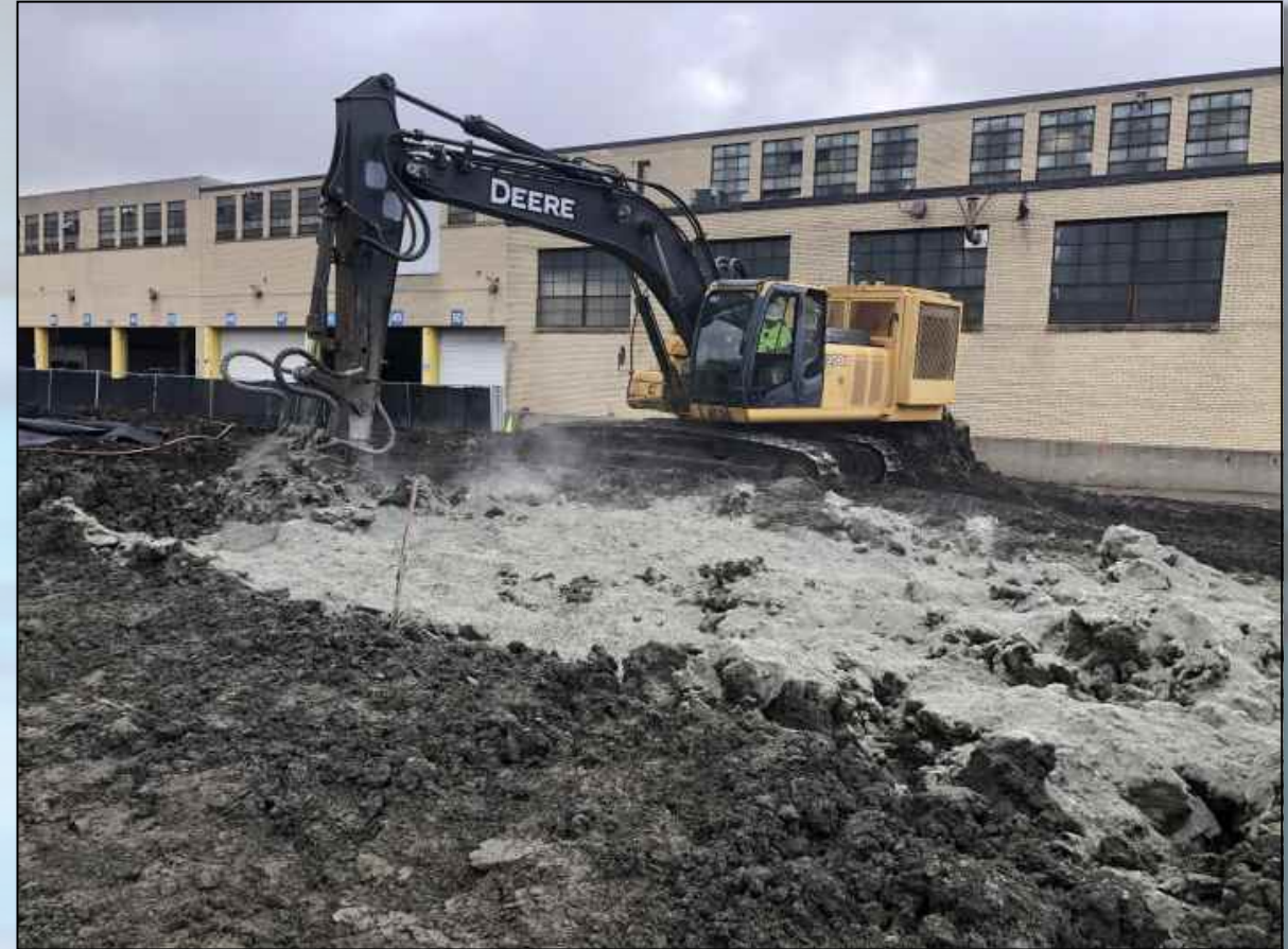
Stabilizing the Top 3 Feet of Soil with Portland Cement
