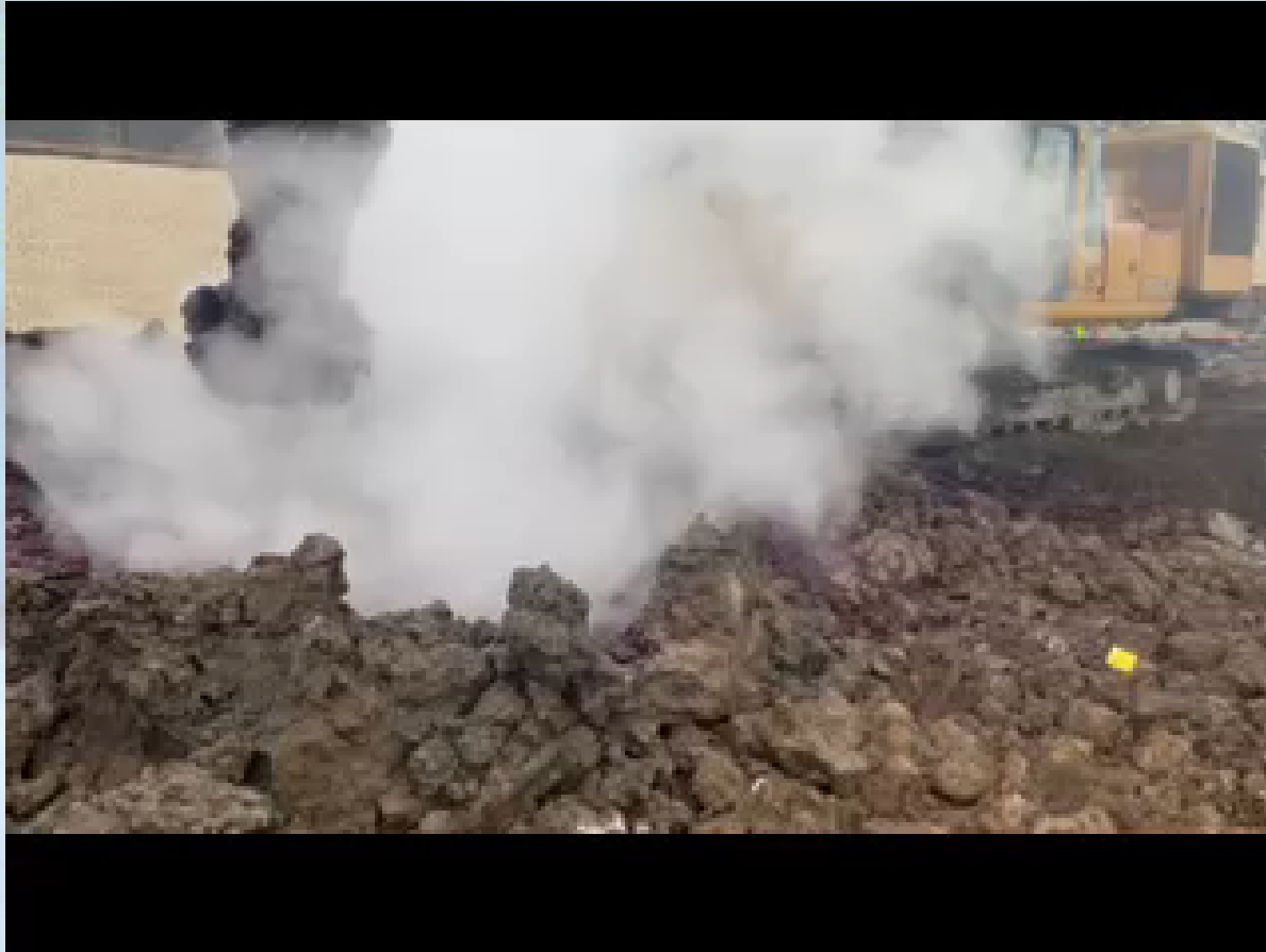
Treating the Top 3 Feet of Soil with Potassium Permanganate
