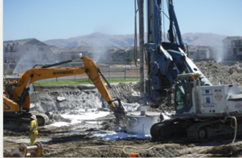
Excavator mounted shroud
