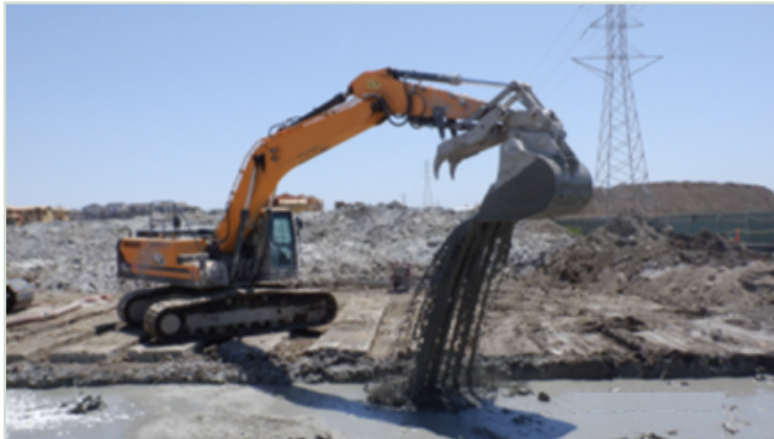
Slurry excavation
