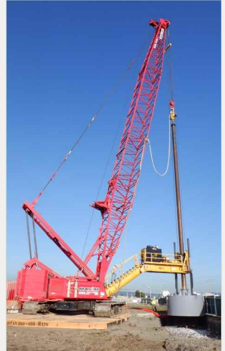
Crane type drill rig
