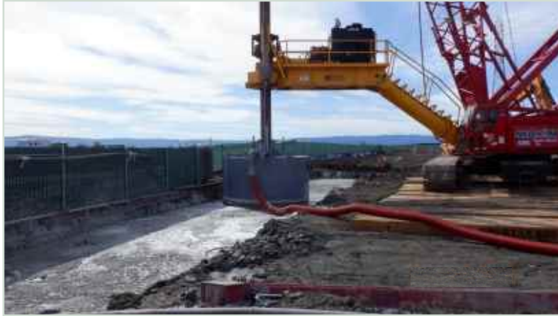
Crane mat use
