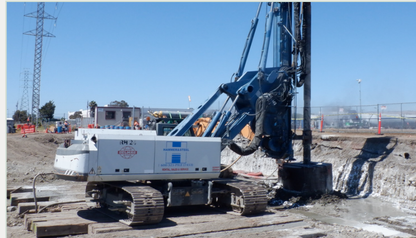
Excavator type drill rig
