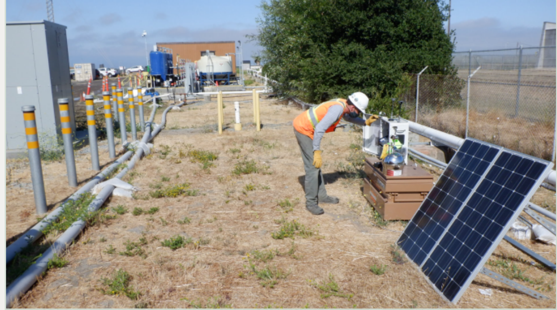
Air Monitoring Station (AMS)
