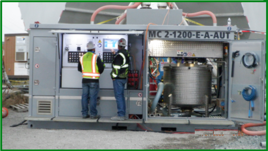
Onsite batch plant
