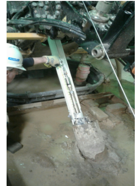
Surveying of completed heater casing using DeviFlex™ tool
