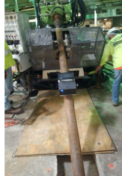
Initial drill casing set-up using DeviAligner™ tool
