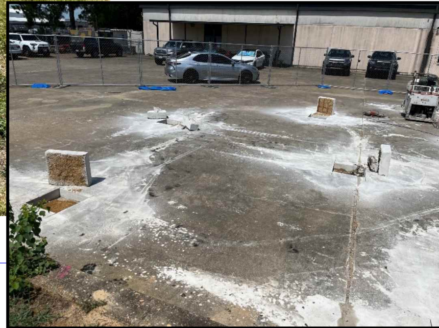
Concrete cores removed from drilling locations on the west side of the TTZ
