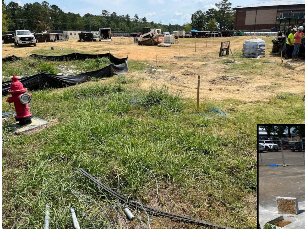
Layout of drilling locations, facing northeast
