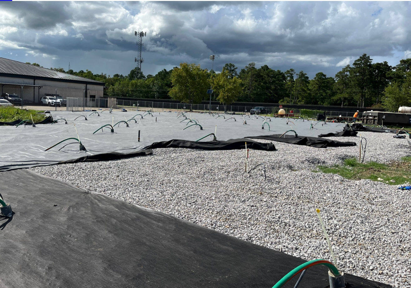
Installation of vapor barrier atop the gravel plenum to facilitate vapor capture, facing northwest
