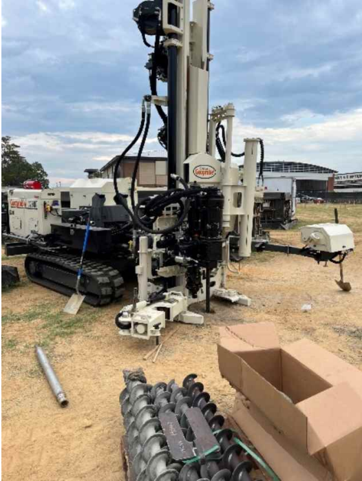
Auger drill rig
