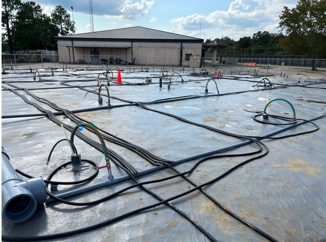
Installation of 3,600 feet of conveyance piping and 26,000 feet of electrical lines, facing west
