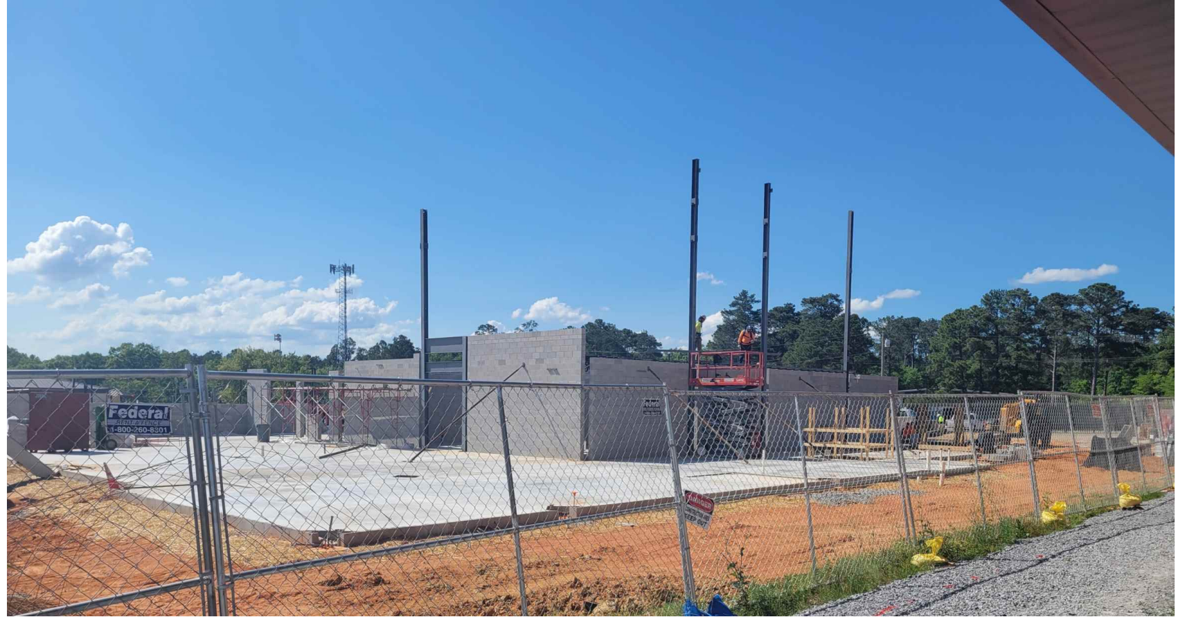
Construction progress as of late April 2024
