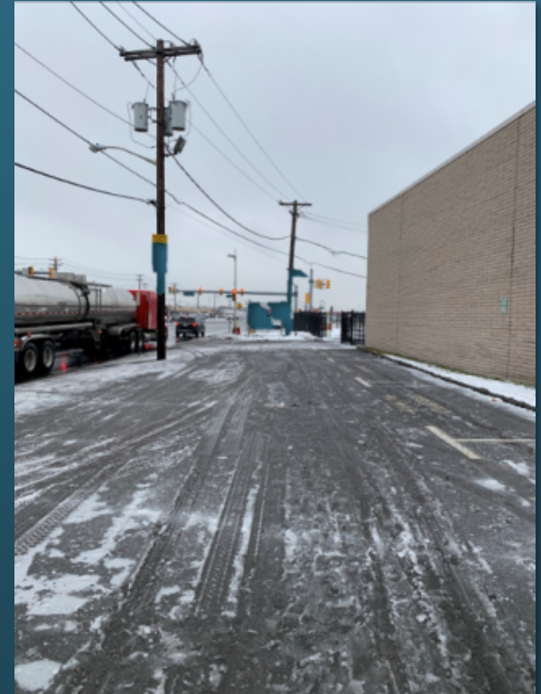
Traffic and overhead electrical power
