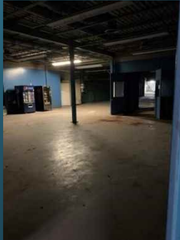
11-foot OH clearance
