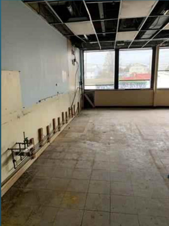
9-foot OH clearance
