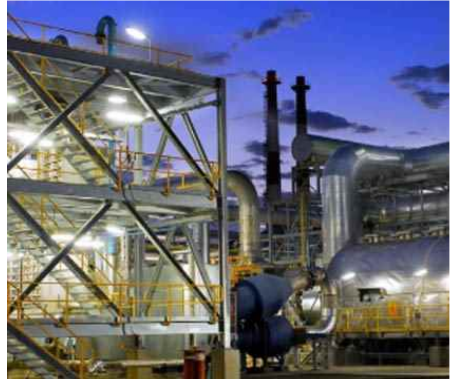
Picture from: Botany Groundwater Cleanup Project - Orica
