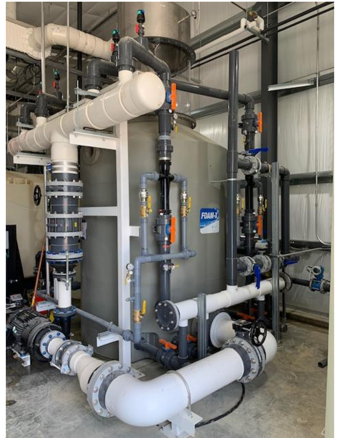
FOAM-X 3000 System for Leachate Treatment Under Construction (US, MO)
