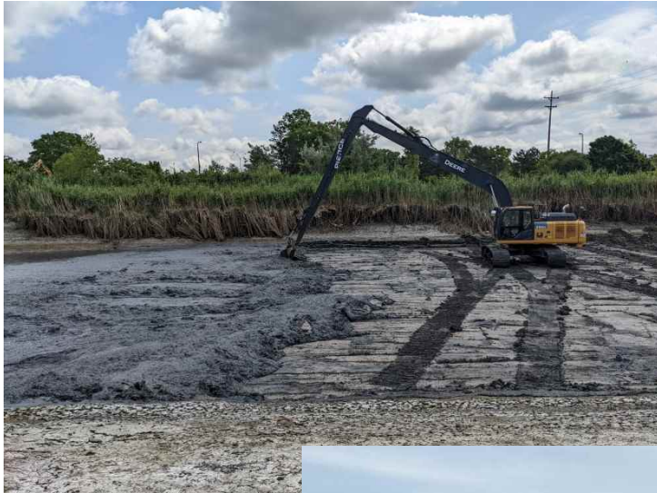
Sediments - Mixing/Stabilization
