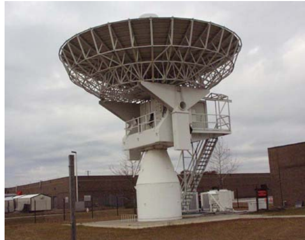
Figure 1. Photograph of an AN/GSC-52A Antenna and Elevated Equipment Room
